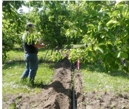
Installation of Solid Set from Hand Lines
