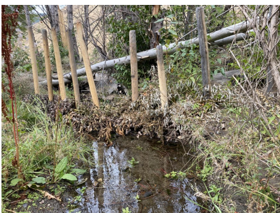
Completed BDA. Photo credit: Trout Unlimited
