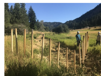
Building the BDA structure
