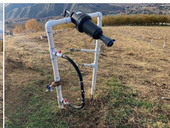
Newly installed water saving pressure reducer and filter for micro and drip irrigation system
