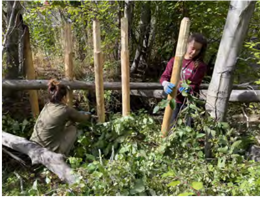
Installing the BDA. Photo credit: Trout Unlimited
