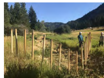
Building the BDA structure
