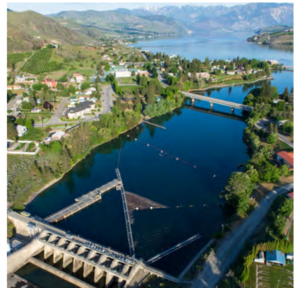
The Chelan Dam generates clean hydropower for the benefit of everyone who lives, works, or plays in Chelan County. Photo by North 40 Productions.
