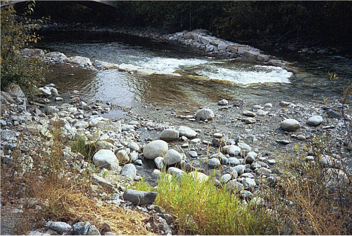
Figure 7-16. View of rock cross vane installed furthest upstream in 2001.
