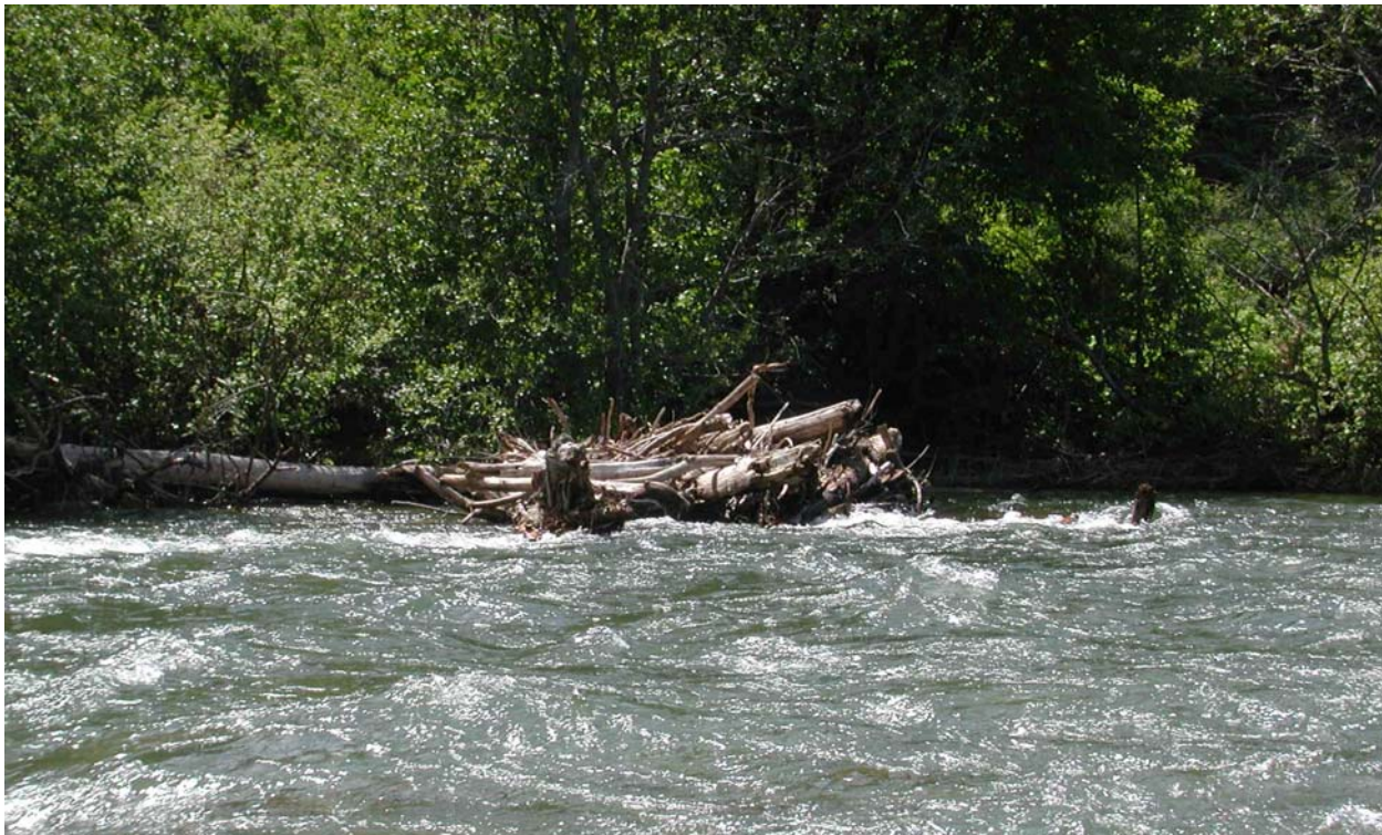
Figure 7-17 One of two engineered log jams installed by the Bureau of Land Management in the lower Entiat River (RM 10.3) during the fall of 2001.
