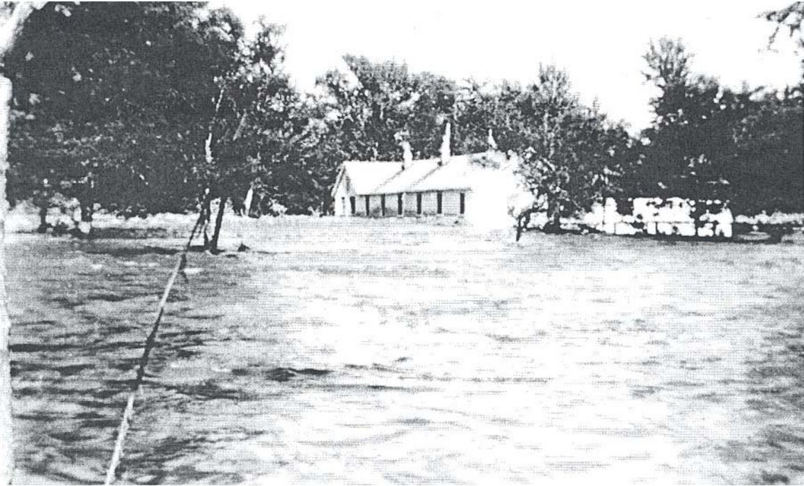
Figure 3-4. View of the 1948 flood, at the Fish Hatchery near RM 7.
