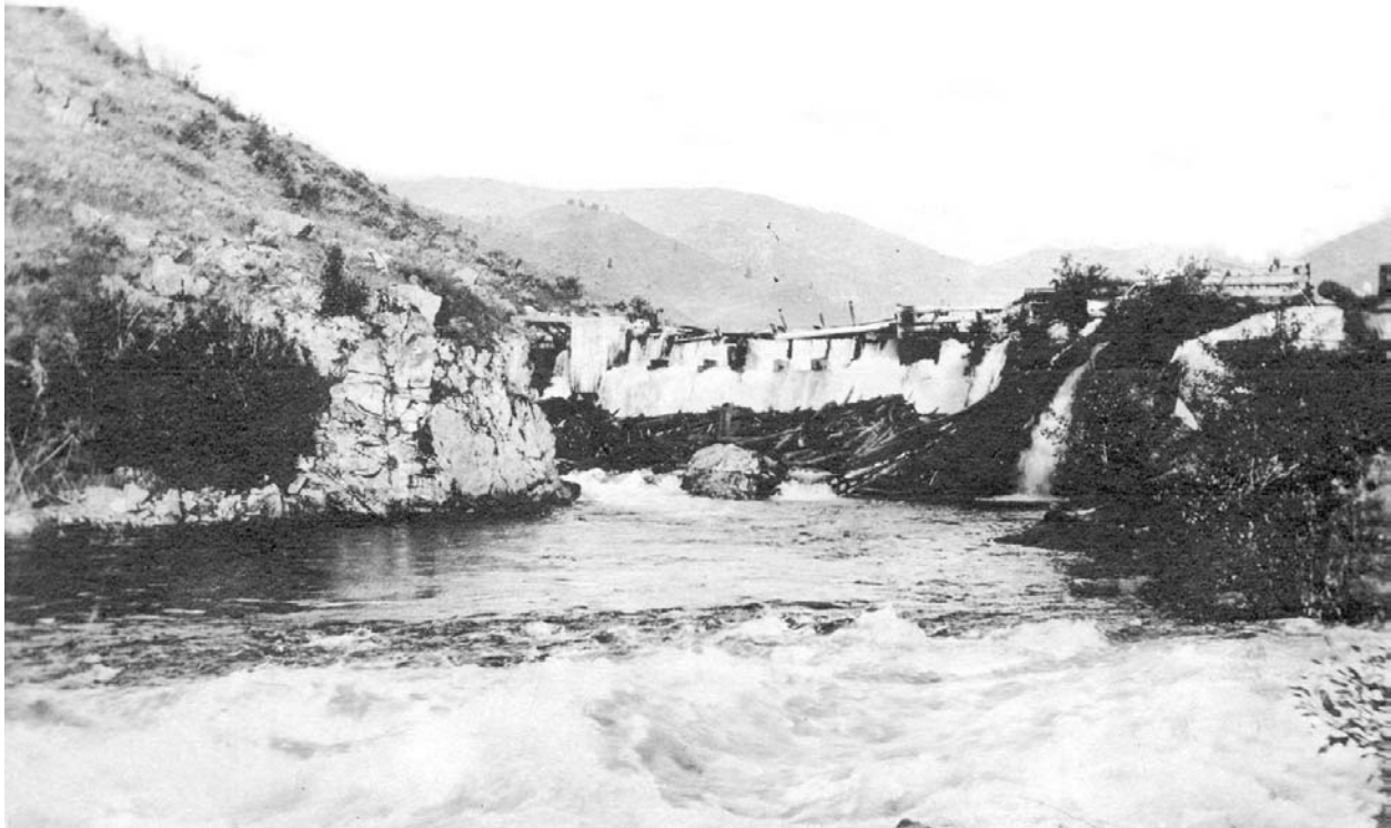
Figure 3-3. Log holding dam constructed at the mouth of the Entiat River, 1898. The Entiat community later removed it to restore fish passage into the Entiat River.
