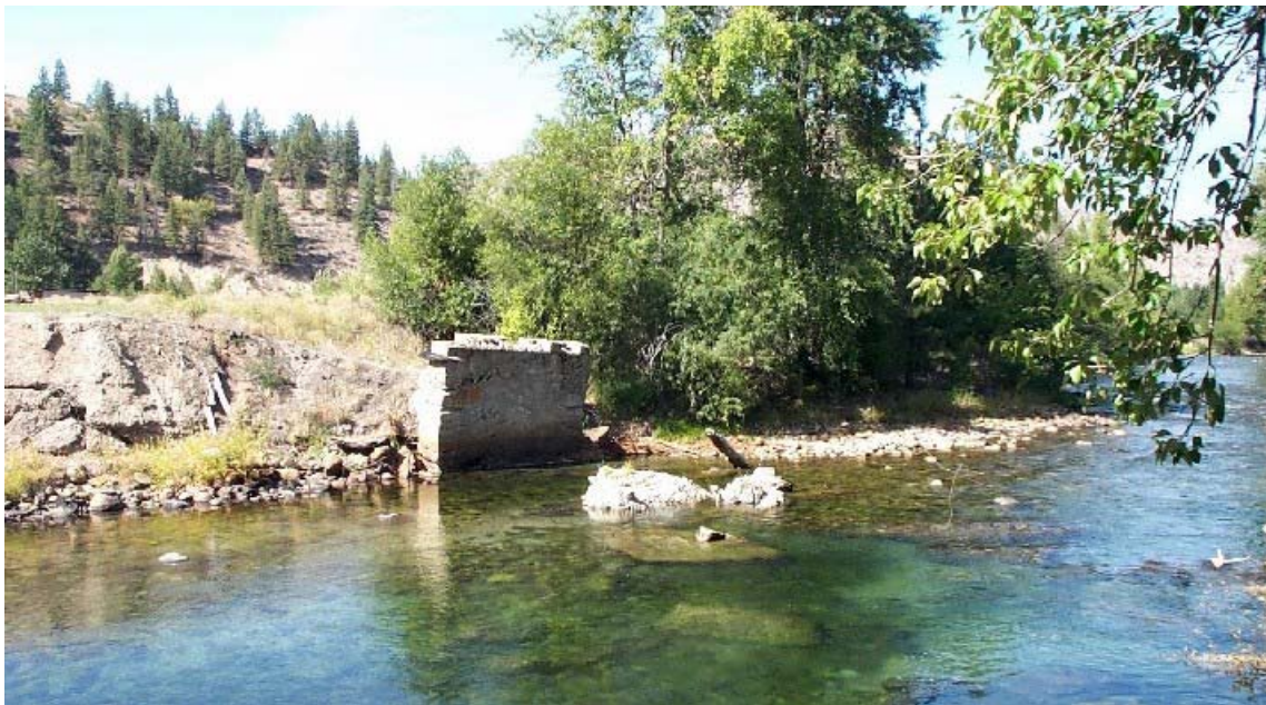
Figure 3-5. Remnant of the Ardenvoir Mill dam, washed out by the 1948 flood.
