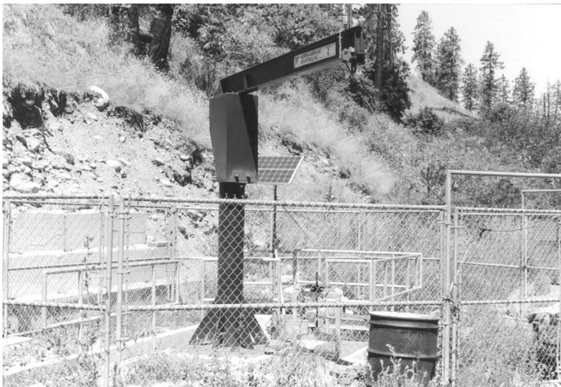
Figure 3-12. General view Hanan-Detwiler fish screen, completed April 1998.
