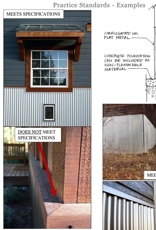
Do not put wood trim on top of metal flashing. Embers can collect on top. Use metal to ensure there are no gaps where embers may enter.
