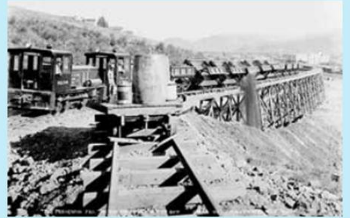
Trestle being back filled
