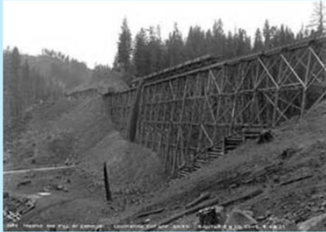
Trestle being back filled
