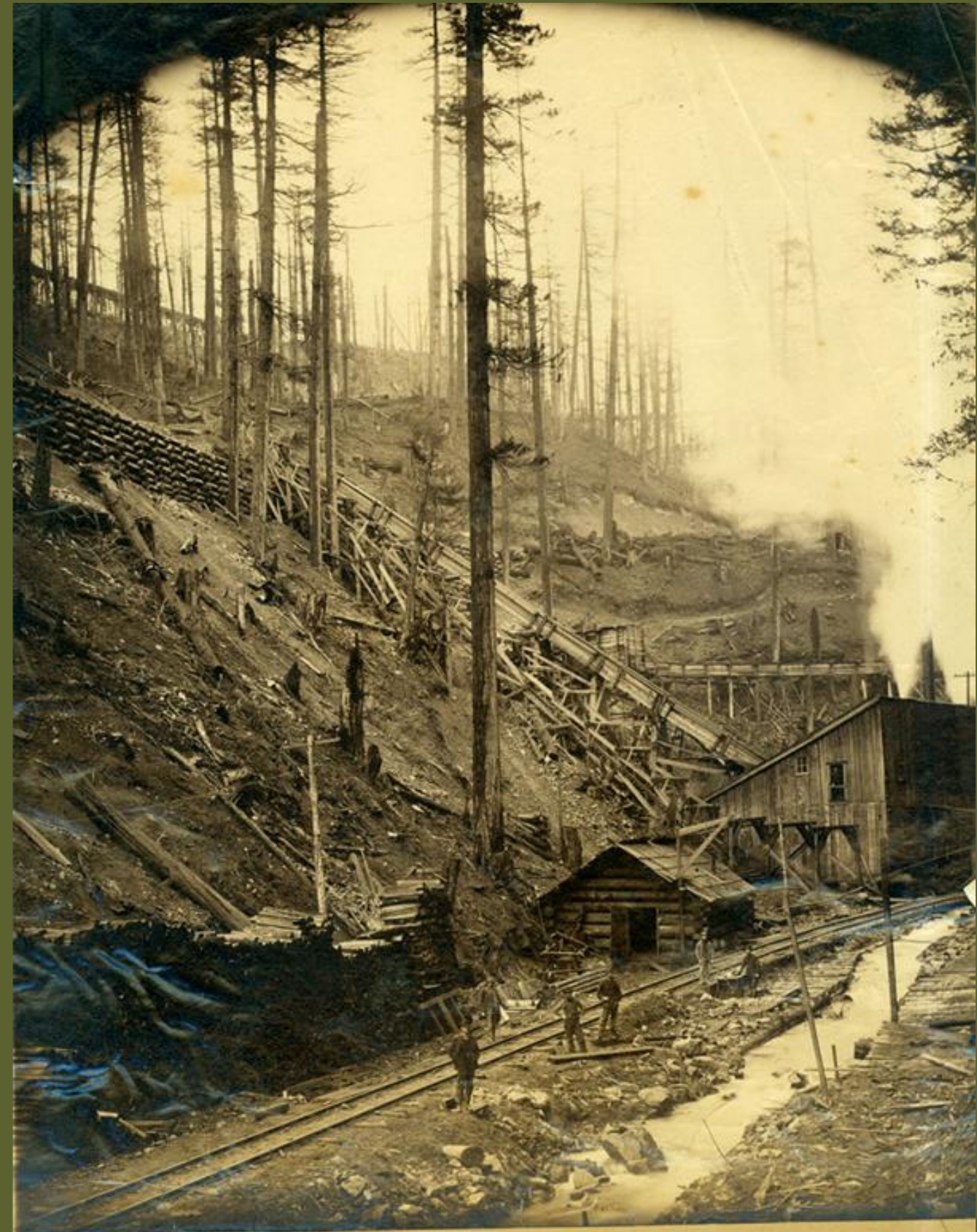
Camp Cr. and Switchbacks, W. Portal Stamped Paper.
