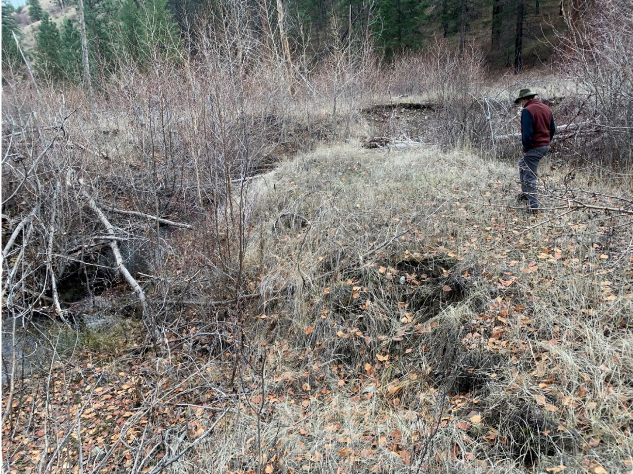
Roaring Creek in November 2021 - Incision of over 2 meters is common within the project area
