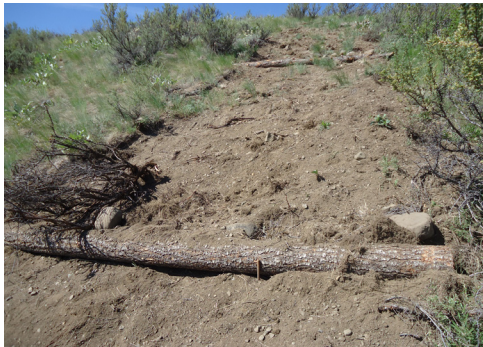
Water bars or simple log check-dams can slow erosion on steep, loose slopes.
