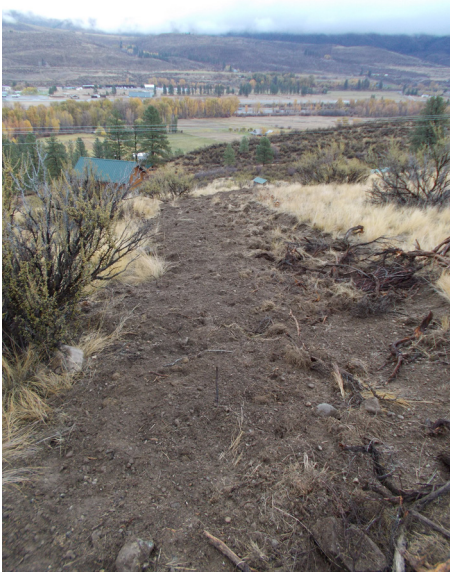
A fireline with removed material pulled back onto the disturbed soil.
