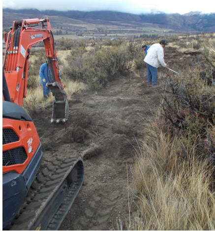
Avoid using heavy equipment like this backhoe if possible.
